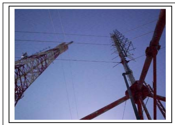
Figure 2. FM Broadcast antenna (right) and TV antenna (left), on top of Tower MOP.
