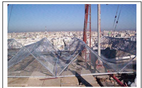
Figure 8. Final shielding structure.
